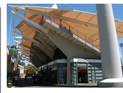
The beams were cast flat on a prestressed concrete base with steel shutters. With six of the beams being heavily reinforced with a 200mm by 200mm slot along the top, the beams required specialist design. Given the enormity of the beams, lifting and positioning posed a challenge. The beams were transported to site on a special heavy trailer, sitting horizontal in the frame during transport.
