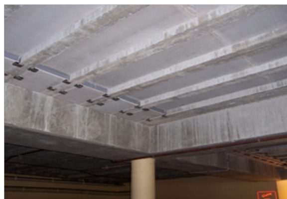
Beam and infill system
