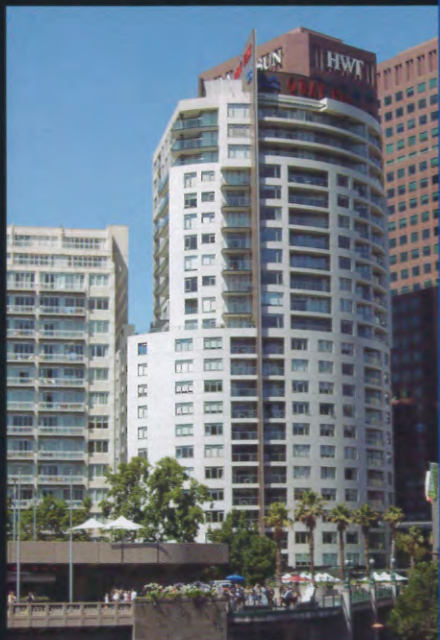
Quay West Melbourne features 330 polished architectural panels, 200 of which are curved.
