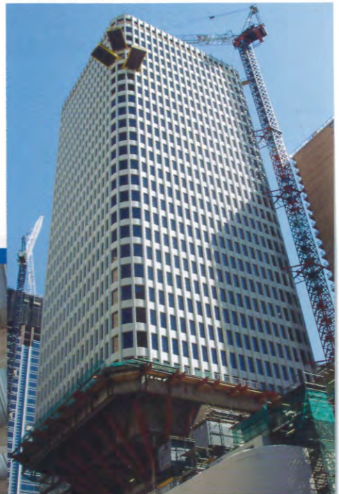
Tower built in record time
