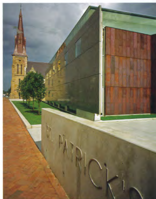
Polished precast panels on the north-south walls contrast beautifully with copper panels on the east-west walls and the magnificent sandstone of the original building. Photo: John Gollings.
