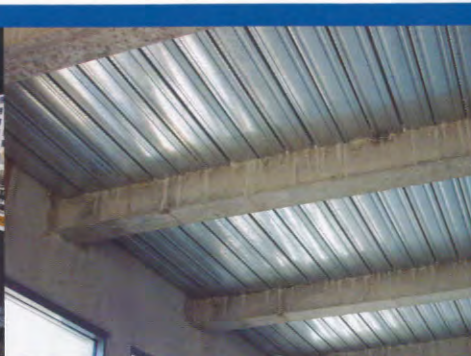
Soffit ready the next day for follow on trades
