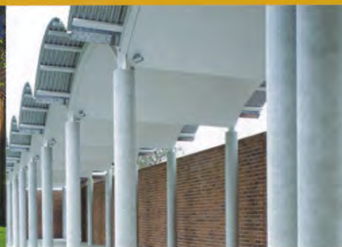
52 off-white precast columns allowed a speedy construction of St Patrick's Cloister area.
