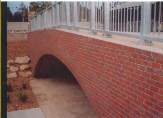
Bricksnaps cast into bridge spandrel façades give a heritage appearance.
