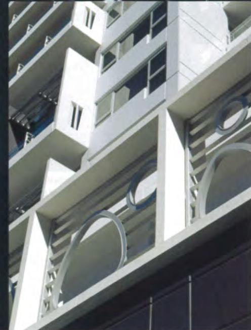
Detail showing balcony blades, spandrels, wall panels and framing units
