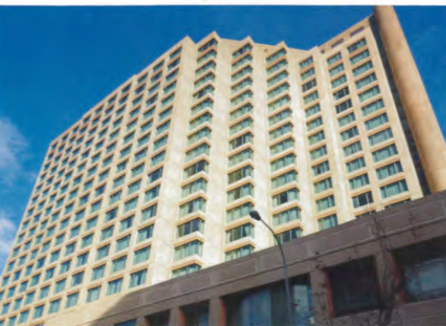
The original Nikko façade featured a combination of sandblasted and painted finishes.
