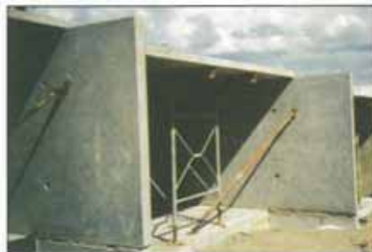
PRECAST PARTY WALLS IN PLACE WITH PRECAST HUMESLAB FLOOR PANELS OVER.
