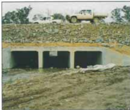
UNITS IN PLACE.
