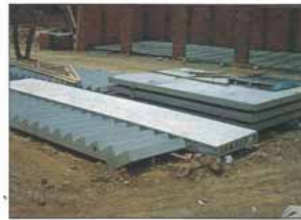
THE PRECAST FAMILY – STAIRS, HOLLOWCORE FLOOR PANELS AND CUSTOM-MADE BALCONY ELEMENTS.
