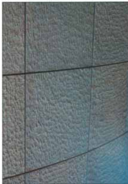
FACADE – OFF-FORM USING TREATED FORMLINER AND RED OXIDE.
