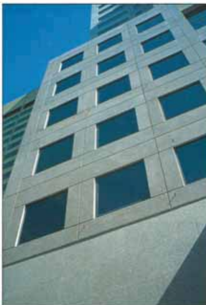
POLISHED FINISH – USING A MIX OF CALCA AND TARANA GRANITE WITH BROWN OXIDE TO TINT THE MATRIX.
