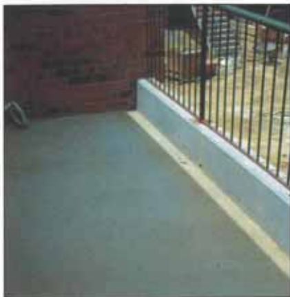
INSTANT SAFETY – PRECAST BALCONY PANEL WITH KERB AND RAILING.
