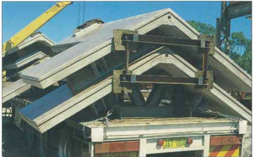
TEMPORARY TRANSPORTATION FRAMES AND PACKING FOR CORNER FACADE UNITS.
