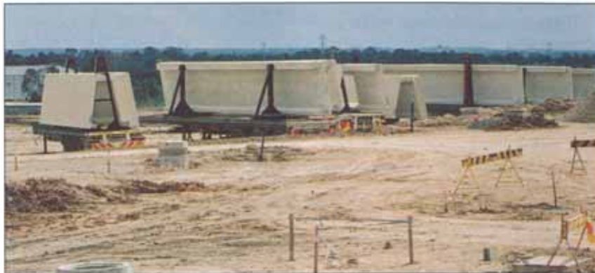
'DROP-TRAILERS' LEFT AT SITE. ENSURES GOOD ERECTION CONTINUITY BUT SPACE NEEDED.
