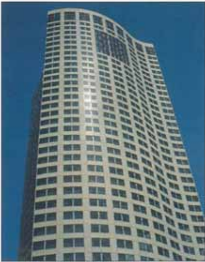
FACADE, ANA HOTEL, THE ROCKS, SYDNEY – A POLISHED, RECONSTRUCTED GRANITE FINISH
