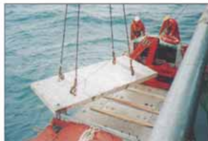
ANTARCTIC SUPPLY VESSEL TRANSFERRING PRECAST PANELS TO BARGE
