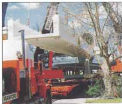
ERECTION OF 93-TONNE PRECAST BRIDGE DECK
