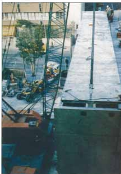
TEE UNITS BEING PLACED, ABC STUDIOS, ULTIMO
