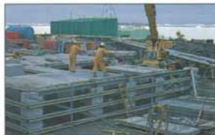
PRECAST CONCRETE FLOOR PANELS AT DAVIS BASE, ANTARCTICA
