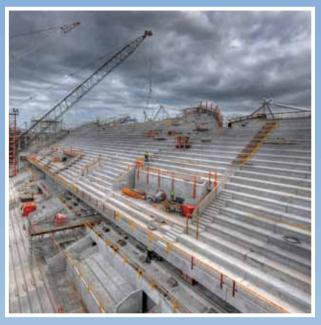
The project also incorporates some 20,000 square metres of hollowcore flooring, a job that required strict attention to detail to ensure that the integrity of each level was retained.
