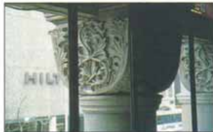
ARCHITECTURAL DETAIL – COLUMN CAPITAL RESTORATION OF QVB, SYDNEY
