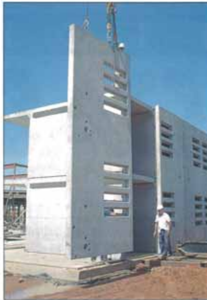
TWO-STOREY REAR WALL BEING LIFTED
