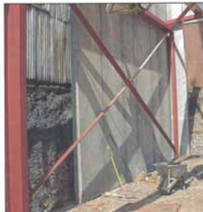
WALL PLACEMENT - NOTE PROXIMITY TO BOUNDARY. FLOOR NOT YET PLACED.
