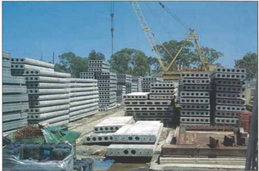
PANELS, STORED AWAITING CONTRACTOR'S DIRECTIONS
