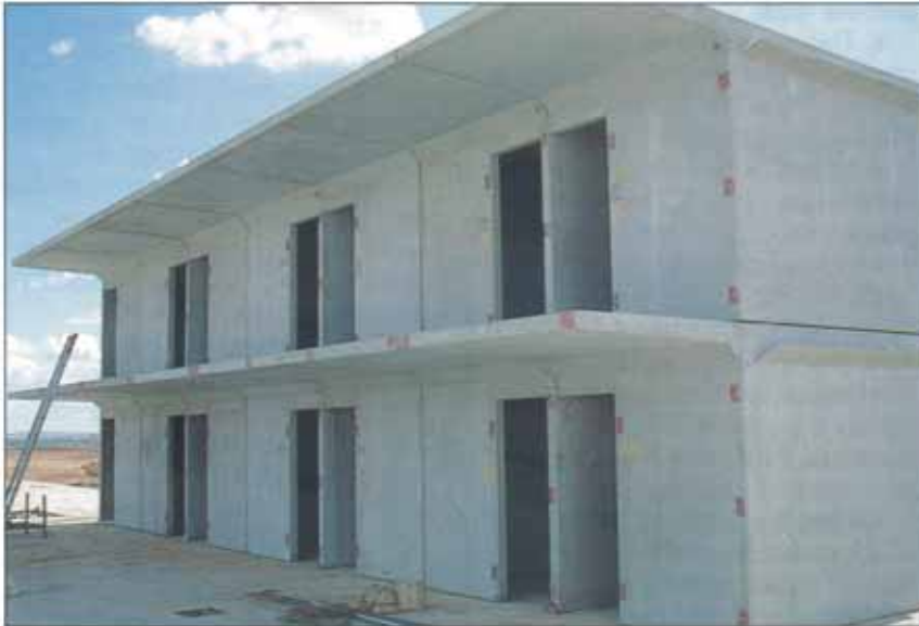
CELL BLOCK – PARTIALLY COMPLETED APPEARANCE
