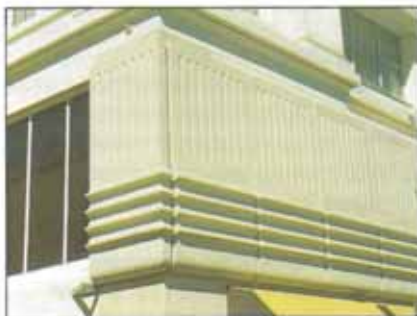
'OVERCLADDING' OF EXISTING FACADE.
