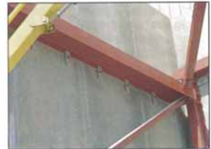
TYPICAL TOP FIXING, TWO CLEATS PER PANEL.
