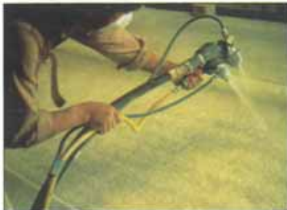
SPRAYING OF GRC
