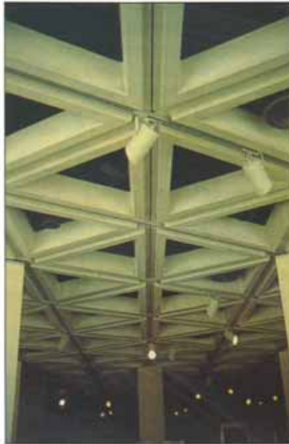
PERMANENT FORMWORK, CEILING DETAIL
