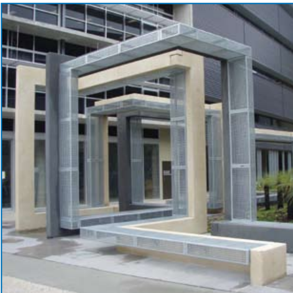
The success of Spun in terms of being a practical piece of art is the result of an equally balanced collaboration between the artist, engineer, architect and precaster.
