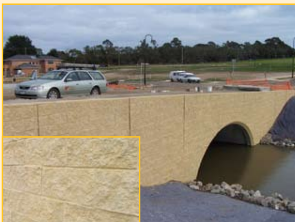
Melbourne's Mt Martha bridge was specified with a 'cream splitface architectural CMU blockwork finish'. Precaster Humes realised that there were significant time and cost savings in casting the bridge sections with a blockwork relief formliner in grey concrete, then staining the moulded surface. The result is one that is indistinguishable from the traditional blockwork that was specified.
