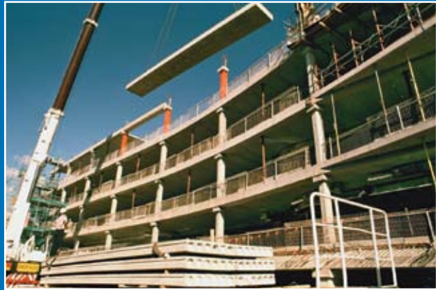
Over 50 hollowcore planks can be placed in a day.
