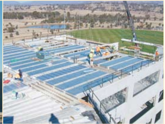
Off-site manufacture means improved site safety because on-site trades are minimised.
