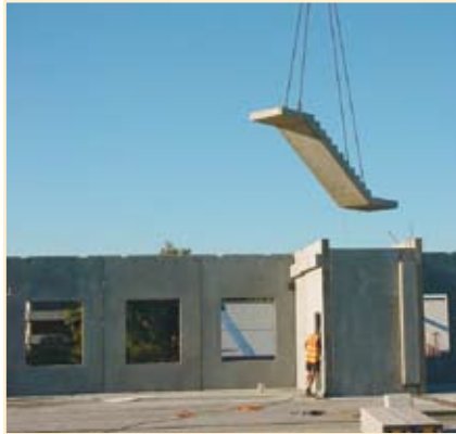
Off-site manufacture means improved site safety because on-site trades are minimised.
