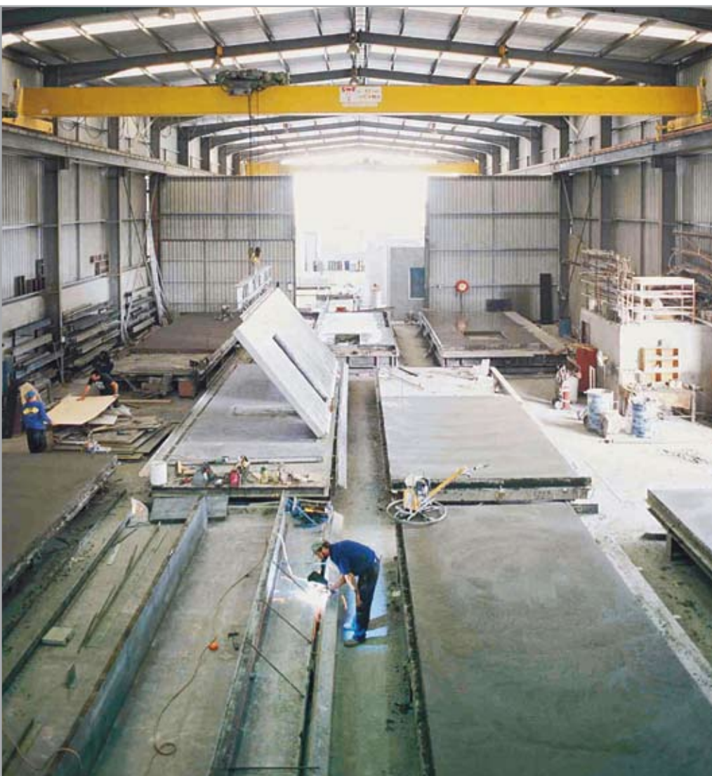
Precast is manufactured under controlled conditions, by specialists in purpose-built factories.
