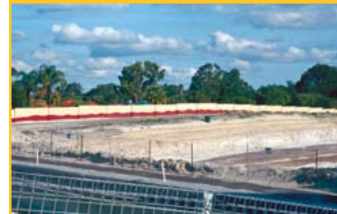
Precast panels provide an effective sound barrier between residential areas and highways.
