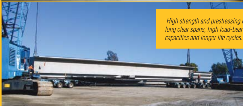
Long clear precast flooring spans mean minimal scaffolding and propping.
