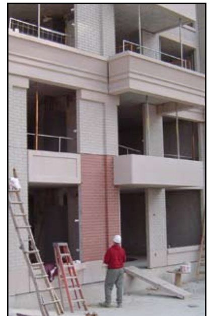
Application of stain transforms moulded precast into brickwork.
