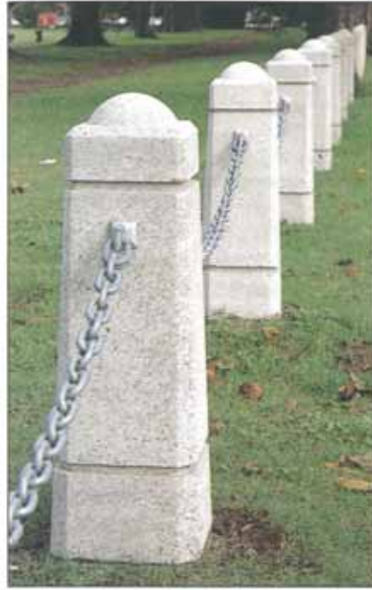
BOLLARDS WITH LIGHT SANDBLASTED FINISH, CENTENNIAL PARK/MOORE PARK TRUST
