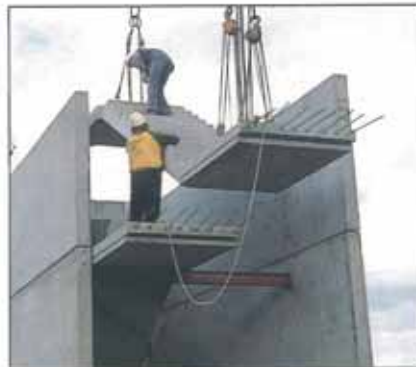
FIGURE 9 CONSTRUCTION SEQUENCE OF THE LIFTSHAFT IN THE ST GEORGE HOSPITAL PROJECT
