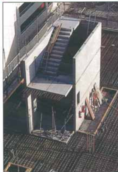
FIGURE 10 CONSTRUCTION SEQUENCE OF THE STAIRWELL IN THE ST GEORGE HOSPITAL PROJECT
