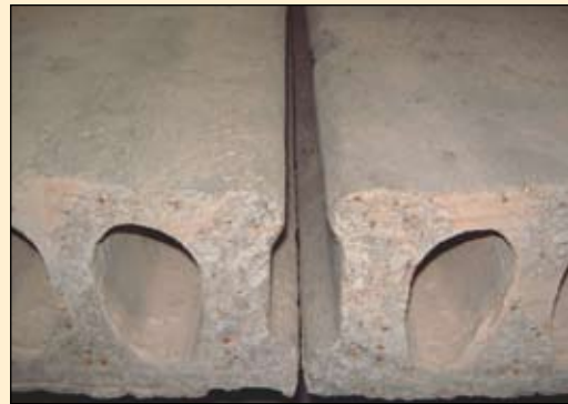
Figure 7: Transverse joint of the hollowcore slabs
