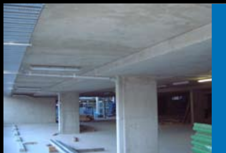
A level soffit aids the even spread of lighting
