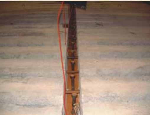
Figure 6: Longitudinal joint with pre-welded headed shear studs
