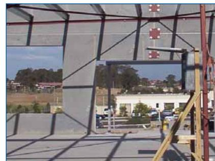
Precast walls in the new KFC Richmond include architectural recesses, penetrations for mechanical equipment, connection points for structural steel and connection points for adjoining panels.
