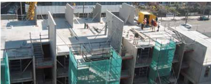
*Division walls being rapidly erected on a completed precast floor of Metro Village.*
