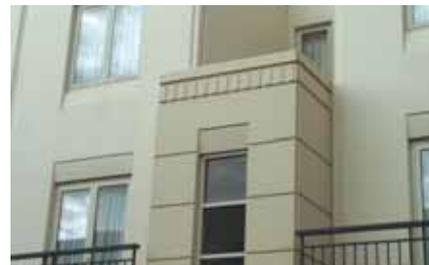
*Design flexibility of precast as exhibited at Balmoral St, Prahran Vic. This apartment block has a number of design features including dummy grooves, projections, ornate corbels and splayed window sills.*
