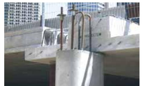
Fig 2: Details of innovative connection in Exhibition Halls between precast beams, columns and floor panels).
