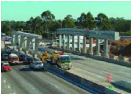
Precast substructure - ready for girders
