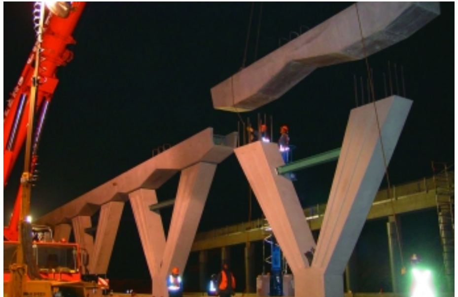
Precast headstocks being erected on Y-shape pier columns
