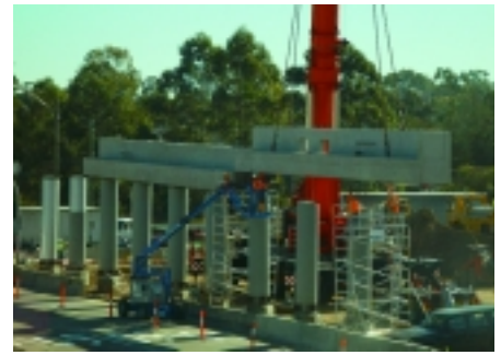
Erection of abutment headstocks.
