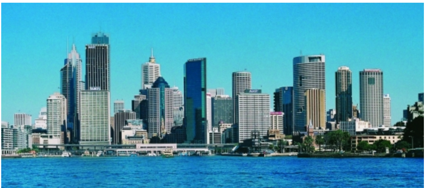
Figure 1. Sydney building facades have various thermal sensitivities. The least sensitive have concrete or GRC facades with shaded windows. Some of the more sensitive unshaded fully glazed facades have low energy star ratings and could become unleaseable if a minimum energy rating of 3 stars were required by prospective tenants. Photographs by E. L. Harkness
