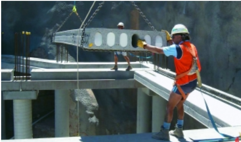
Hollowcore planks deliver strength and fire rating with up to 45% less material plus savings in structure dead load and transport costs.
