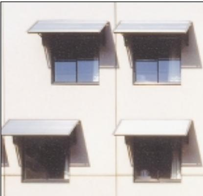
Honed reconstructed stone finished panels with staggered window layout
