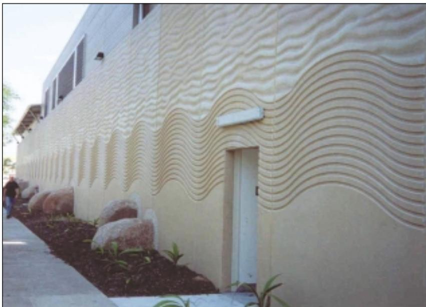
Tidal Wall formed by precast coloured acid-washed 6m high panels and sculptured boulders
