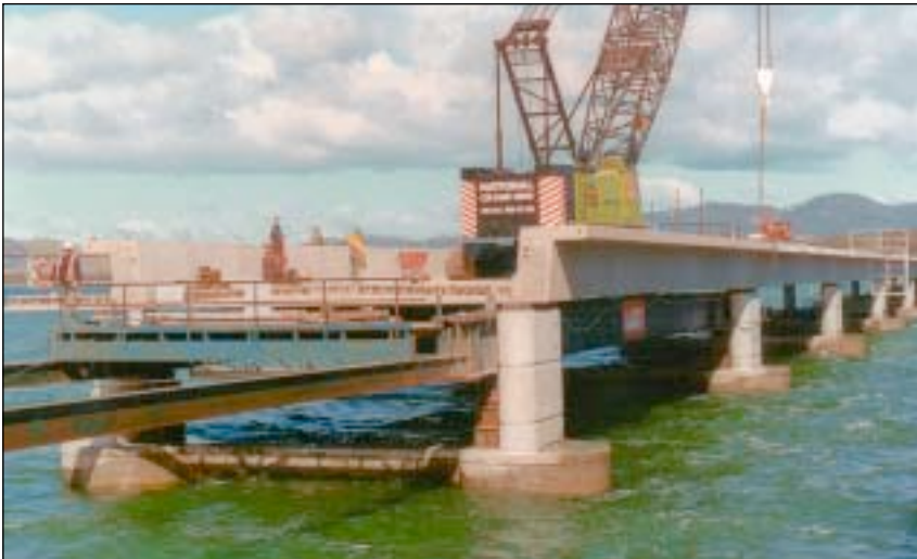
(above) A massive 150 tonne capacity crawler crane sits atop the completed span. The crane was used to lift ten precast segments making up the next span onto steel falsework. Each segment weighed up to 46 tonnes.
