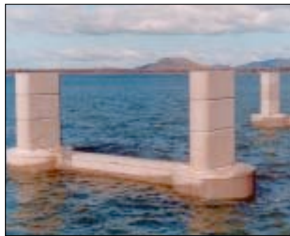
View of substructure. Precast pier units were stressed vertically to pilecaps
