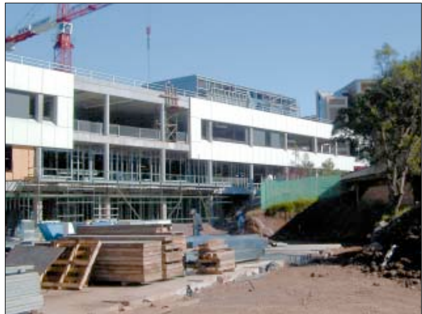
Lightweight GRC facade panels being installed at Sutherland Hospital, Sydney
