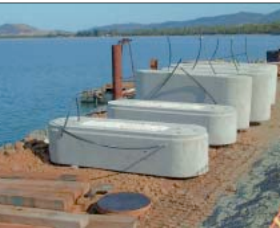
View of hollow precast pier column units. These were match-cast vertically in factory conditions.
