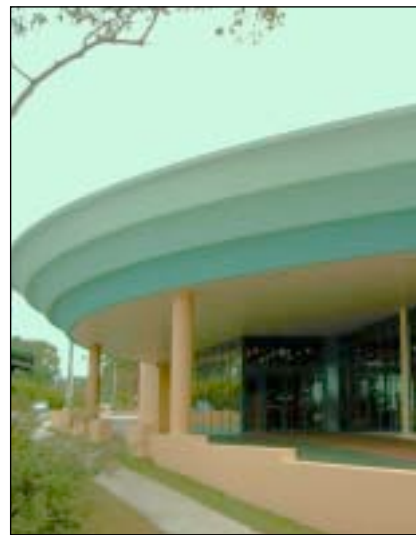
Curved GRC fascia panels provide aesthetic definition to Club foyer entry
