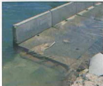
PRECAST UNIT DELIVERED ADJACENT TO FINAL PLACEMENT POSITION.
