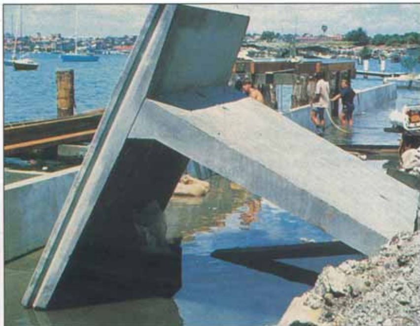
PRECAST UNIT DELIVERED ADJACENT TO FINAL PLACEMENT POSITION.
