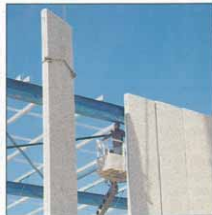
ERECTION OF 12-m-HIGH, WATER-WASHED, EXPOSED-AGGREGATE HOLLOW CORE PANELS BY THREE WAY CONSTRUCTION.
