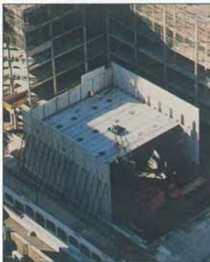
ERECTION OF 12-m-HIGH, WATER-WASHED, EXPOSED-AGGREGATE HOLLOW CORE PANELS BY THREE WAY CONSTRUCTION.
