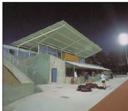
Hockey Stadium at Curtin University featuring precast wall panels up to 6.5 m width.
