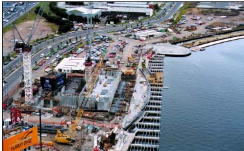
(above) Sections A and B of the car park for Yarra's Edge building No.3. Note the large spans (12.3 m) of hollow core planks providing high efficiency in space utilisation (below) Aerial view of Yarra's Edge building No.3 carpark in construction. A 31 level tower will rise above the five level above-ground carpark
