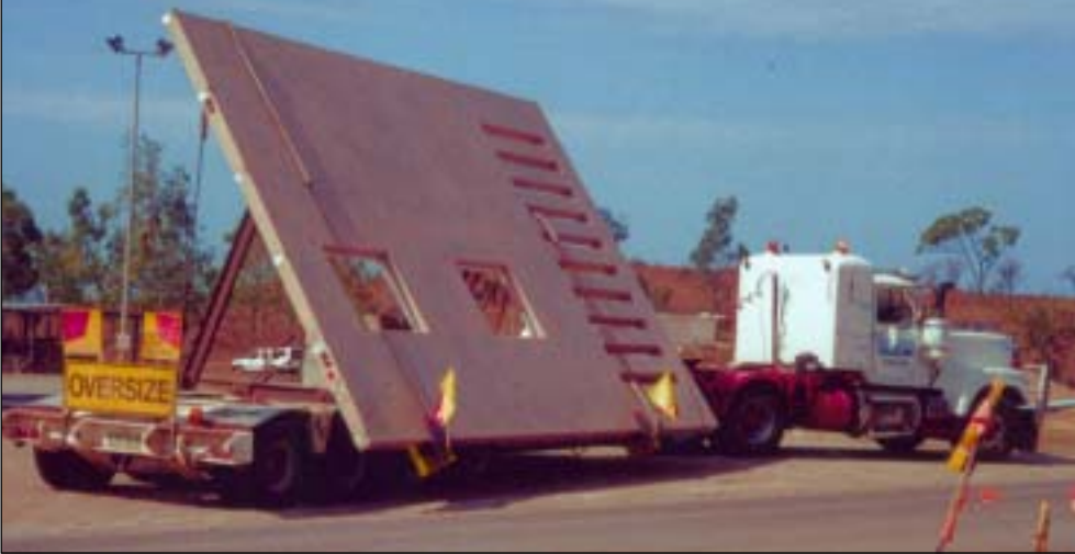
Customised counterweighted transportation rig for overdimensional panels – 11 m long and 5 m wide weighing up to 16 tonnes each
