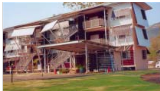
Completed standard 18-unit building with L-shaped floor configuration
