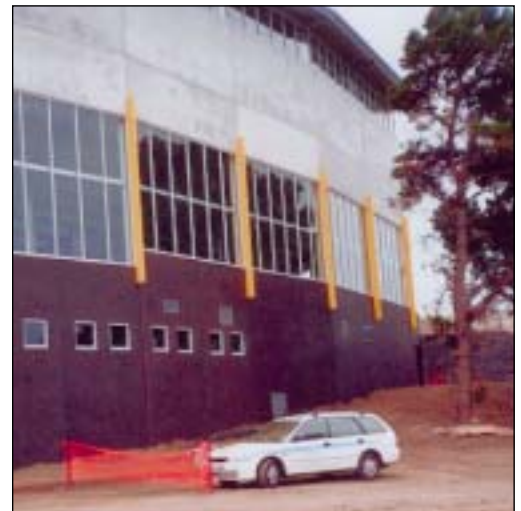
Rear view of Southern Stand showing 6.5 m height coloured precast wall panels
