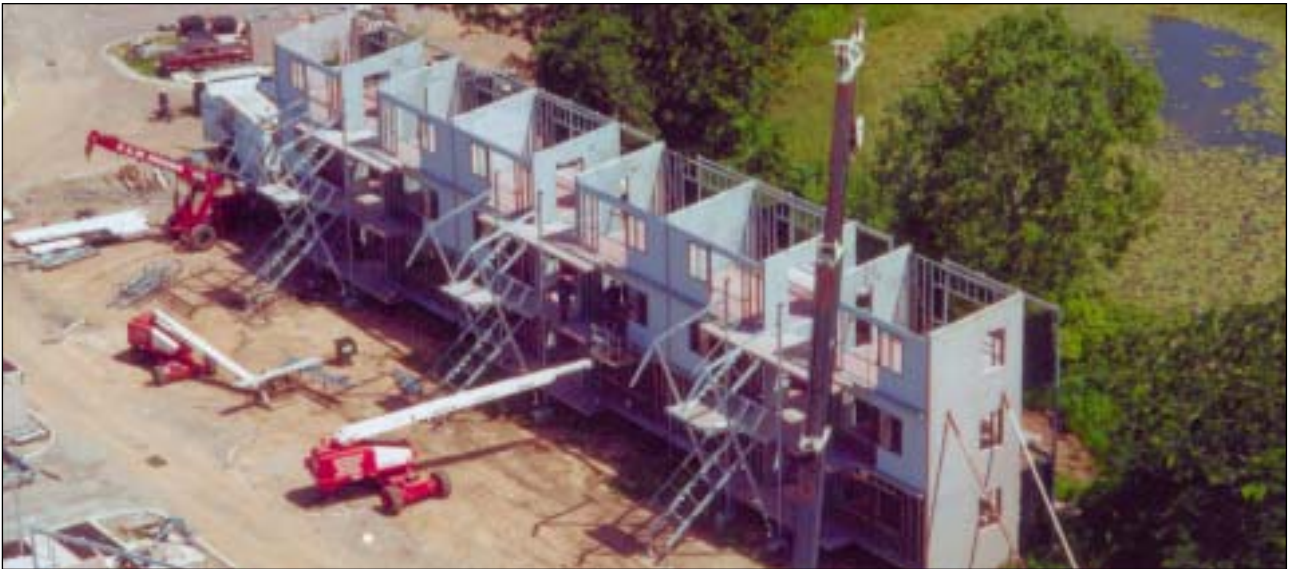
Partially erected 18-unit building with rectangular polished floors
