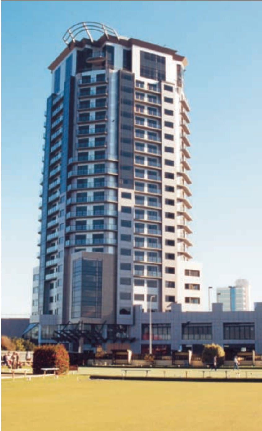
Spencer on Byron completed structure
