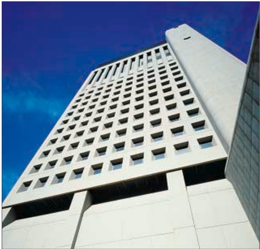
Commonwealth Bank Building, Sydney – an example of a high quality, durable veneered facade
