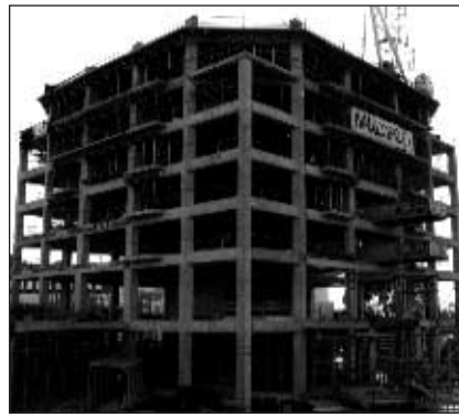
Spencer on Byron building under construction
