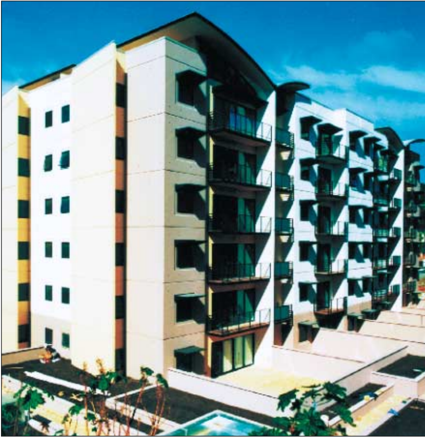
Stage 1 of Mounts Bay Village, Perth designed as a fully precast building (above) and the front view of typical 2.9 m high x 5 m wide off-form painted external wall panel (right).
