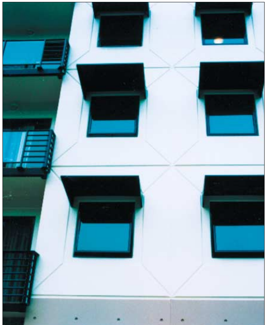
Stage 1 of Mounts Bay Village, Perth designed as a fully precast building (above) and the front view of typical 2.9 m high x 5 m wide off-form painted external wall panel (right).
