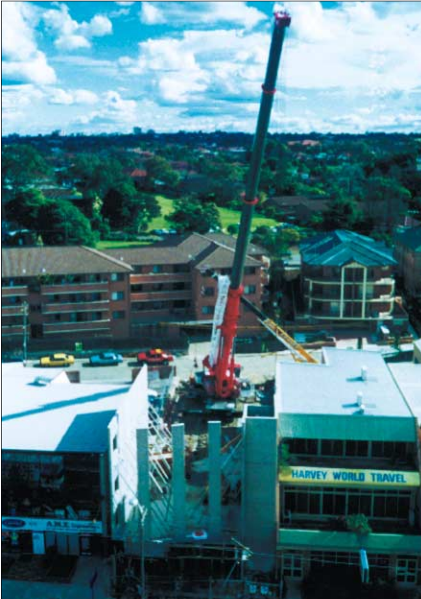
Aerial view of wall panel erection at narrow Rockdale site.
