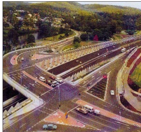
Elevation of multi-hued panels after erection (above) and an aerial view of Nerang-Broadbeach Road featuring some 362 precast noise barrier panels (right)
