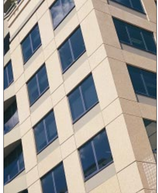
High-rise office building clad with high-quality polished facade panels providing Class 2 finish – the best the precast industry can produce
