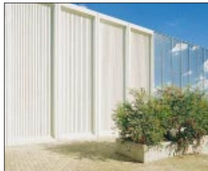
Top quality Class 2 off-form finish in industrial building representative of best industry practice
