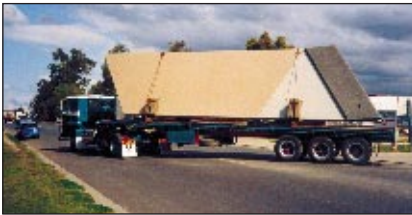
Panels in storage at precaster's yard awaiting delivery (above) and a 6.2 m x 3 m precast panel being transported from factory (left)
