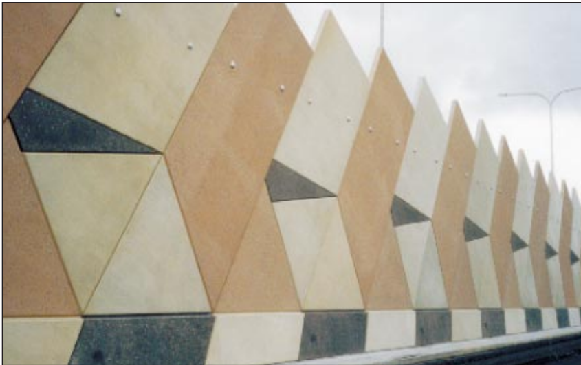
Elevation of multi-hued panels after erection (above) and an aerial view of Nerang-Broadbeach Road featuring some 362 precast noise barrier panels (right)
