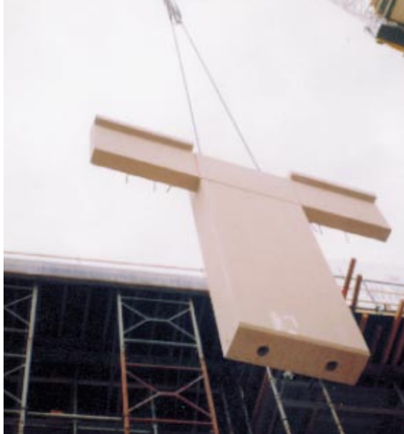
T-shaped precast panel incorporating overhanging sill being hoisted into place
