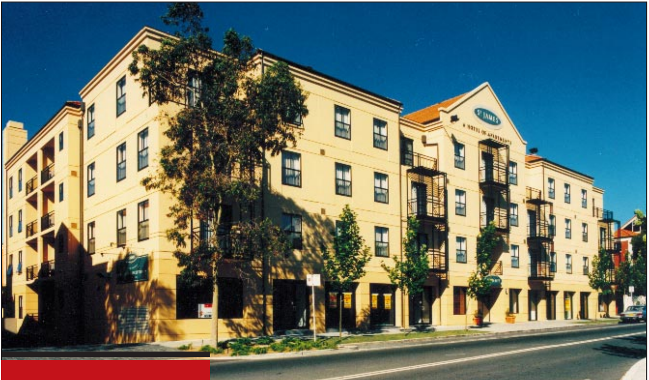
Total precast structure of St James Estate, Northbridge, Perth, WA
