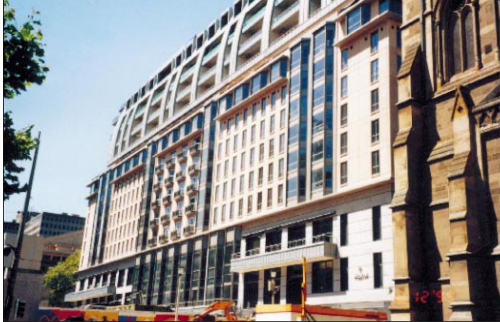
Western elevation of Westin Hotel facing Swanston St, Melbourne
