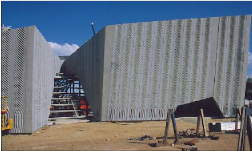
Erection of moulded facade panels. Note asymmetrical design of wall elevations.
