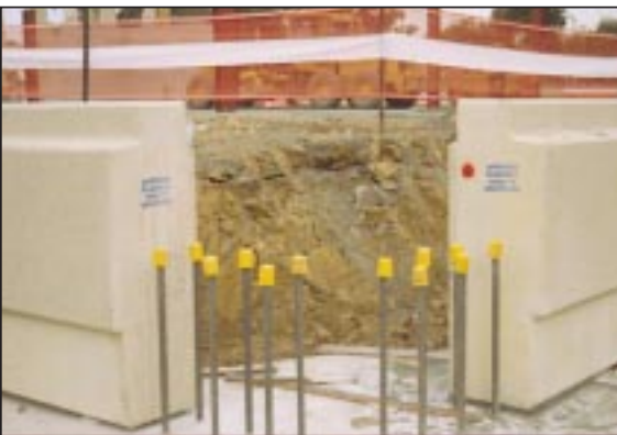
Starter bars for a loadbearing column connection
