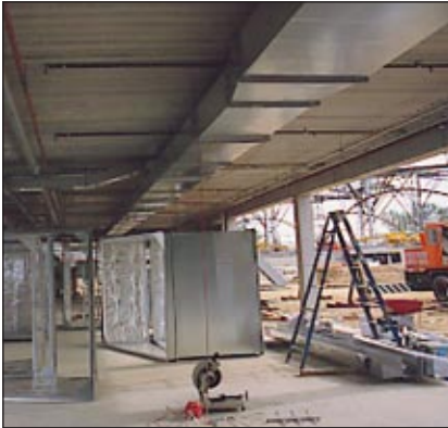
Hollowcore floor panels installed to speed up construction.
