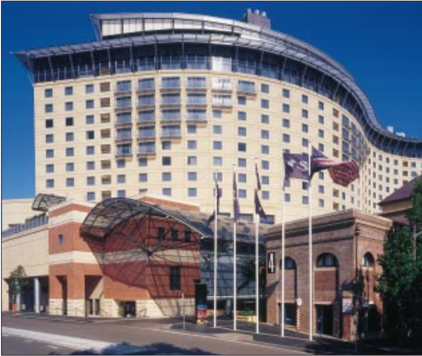
Precast panels on Sydney Hotel/Casino complex using 0.75% yellow oxide
