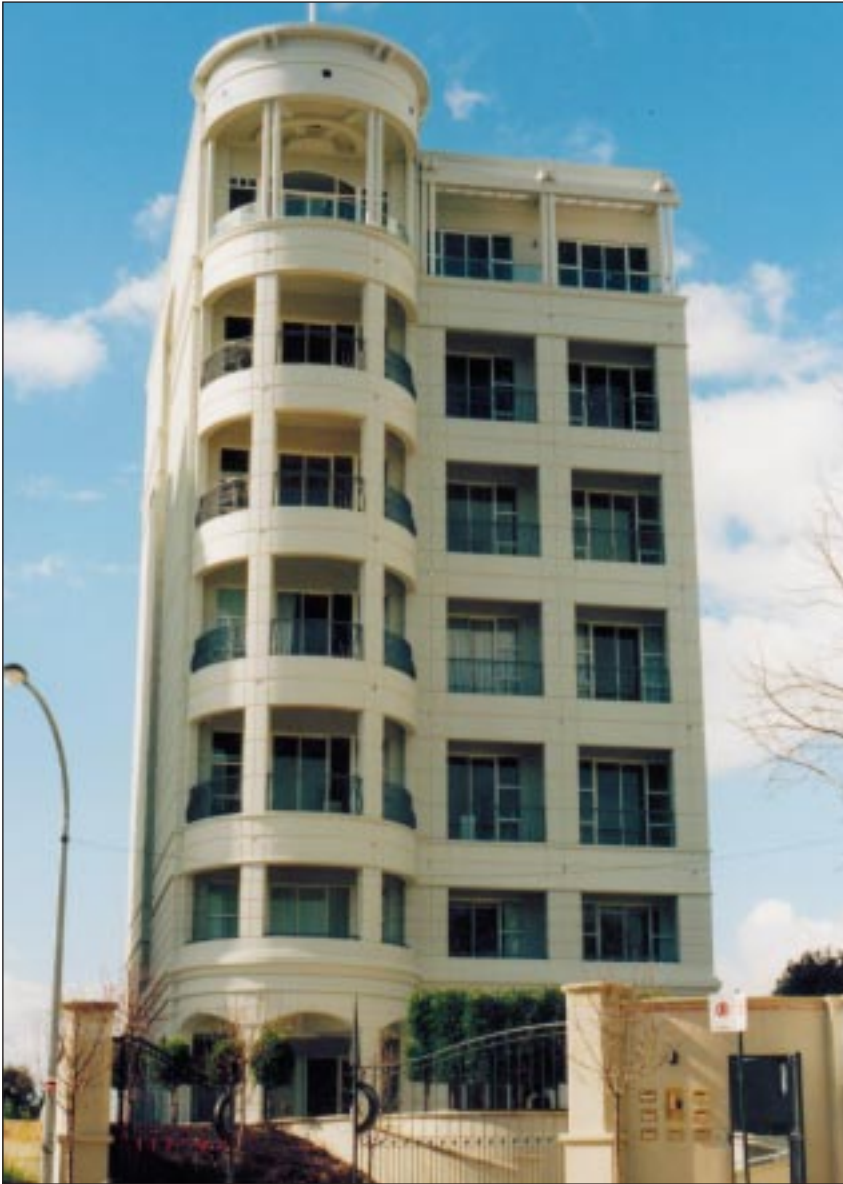
Award winning Goldman Apartments in South Perth built exclusively in factory precast concrete featuring a wide range of precast components including architecturally finished wall spandrels, internal lift shaft wall panels, beams, columns, balcony panels as well as floors
