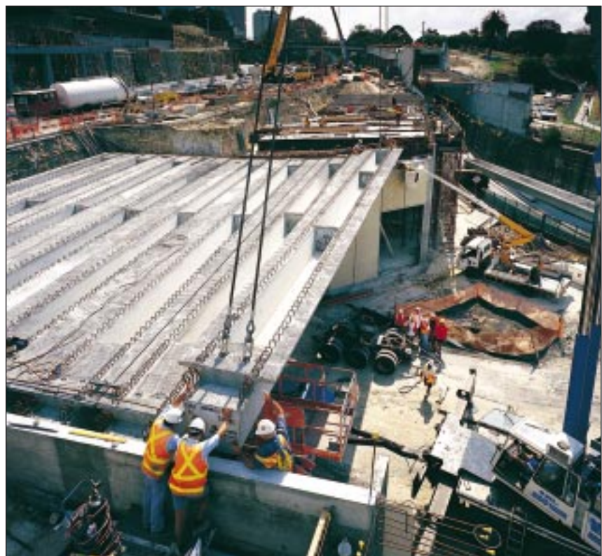
Installation of Super T bridge girders and planks for Landbridge
