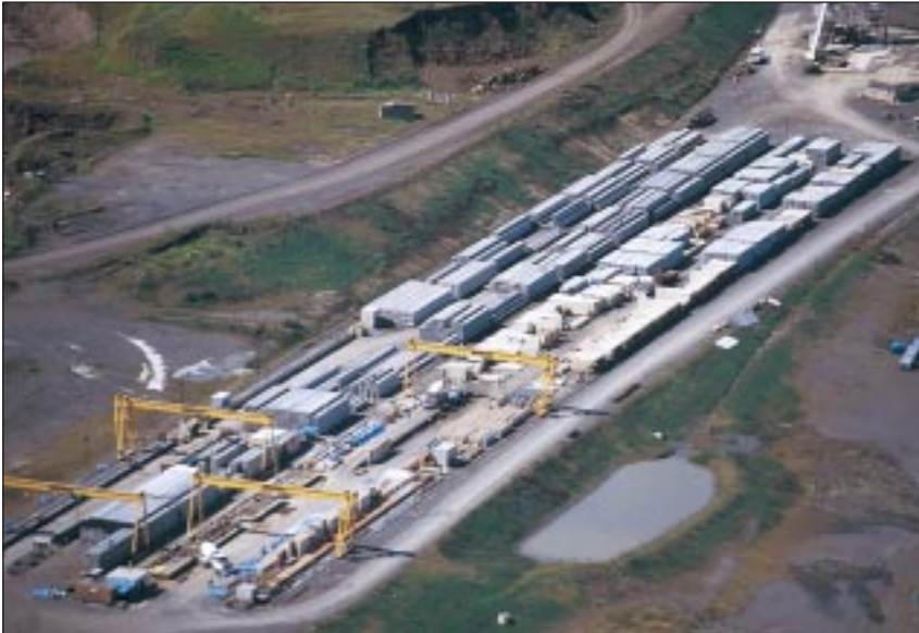
Precast plant for Eastern Distributor at Erskine Park, Western Sydney
