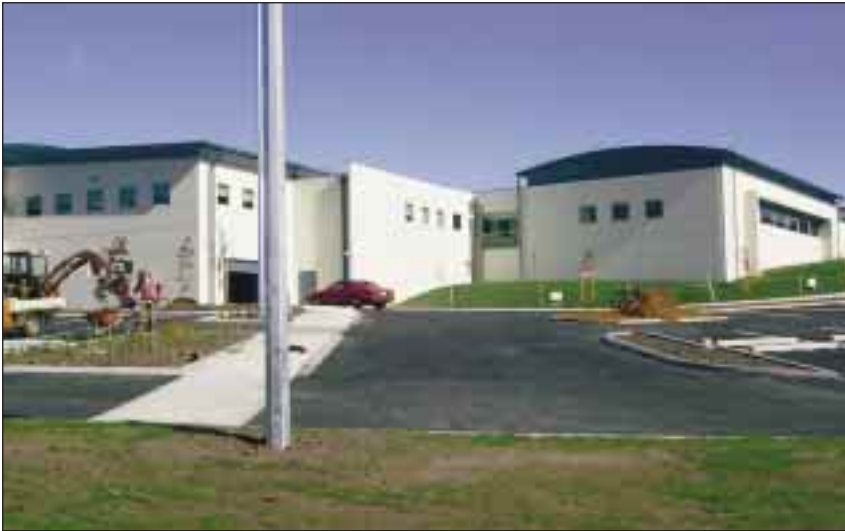
Front elevation of painted precast wall panels in Vodaphone Building Complex shaped load-bearing wall panel on front elevation
