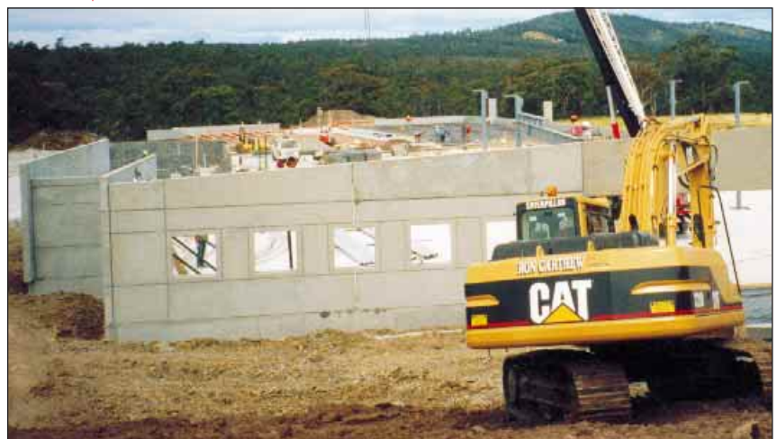
Erection of 6.3 m x 4 m window panels on Vodaphone Building
