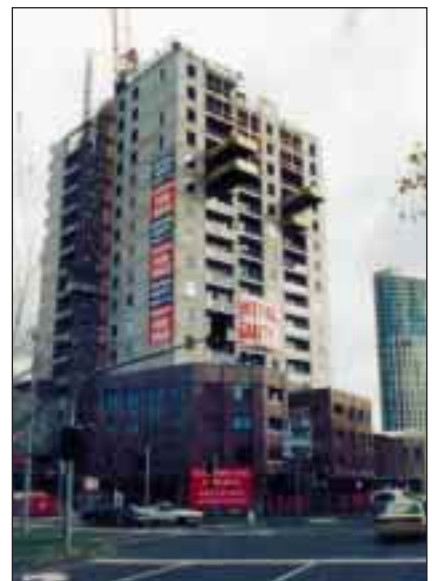
24 Level apartment block, Southbank Condos under construction in Melbourne's Southbank
