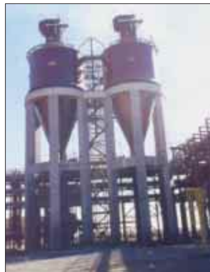
The 1000 tonne copper concentrate bin after installation
