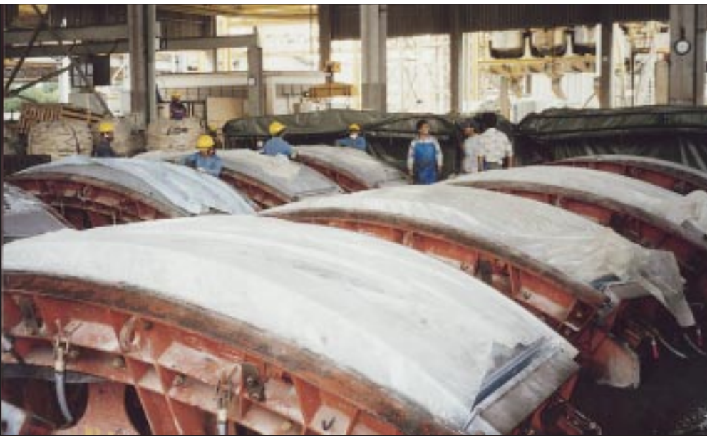
SEGMENTS READY FOR DEMOULDING
