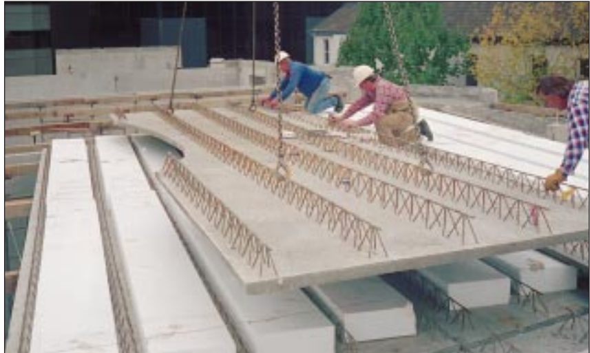
SEMI-PRECAST PANELS BEING PLACED ON SITE
