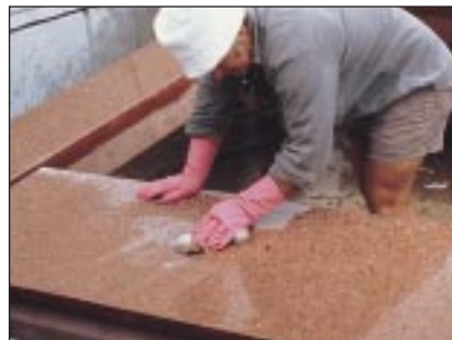
LIGHT ACID CLEANING OF POLISHED PANEL PRIOR TO DELIVERY
