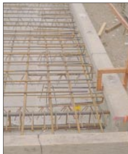
TRANSFLOOR PANELS CONNECTING INTO A LOAD BEARING WALL
