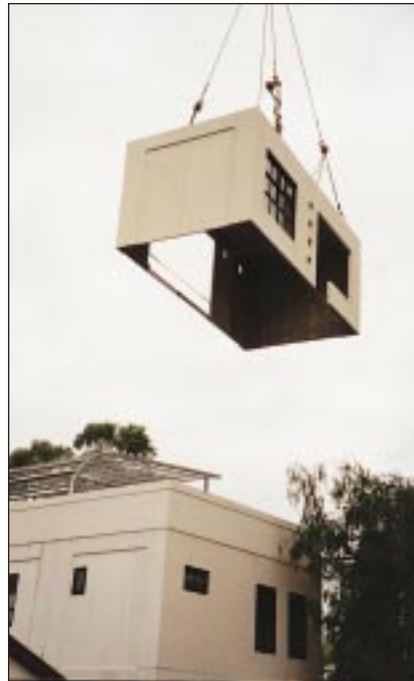
PLACING A TYPICAL MODULE
