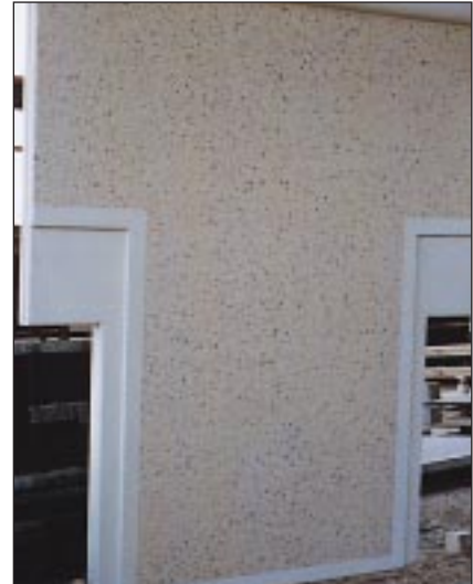
SHOWS BLASTING WITH PROFILED HEAD OF THE PANEL AND SURROUNDS TO WINDOW OPENINGS LEFT SMOOTH OFF-FORM
