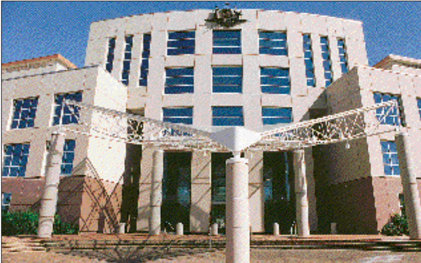
30 000 SQUARE METRES OF SANDBLASTED OFF WHITE PRECAST CONCRETE WAS SUPPLIED TO CLAD THE DEPARTMENT OF FOREIGN AFFAIRS AND TRADE BUILDING IN CANBERRA
