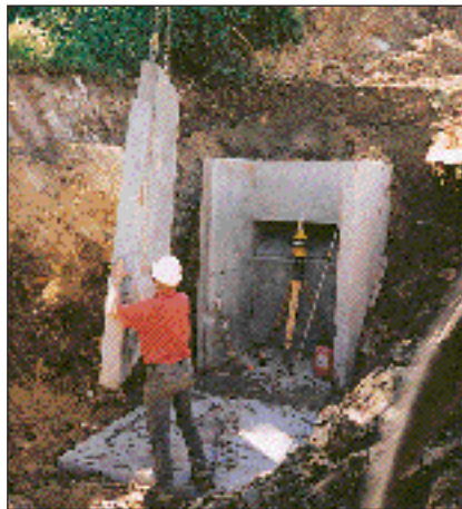
PLACING PRECAST CONCRETE MODULAR WALL PANELS; NOTE WORKFORCE CONTENT.
