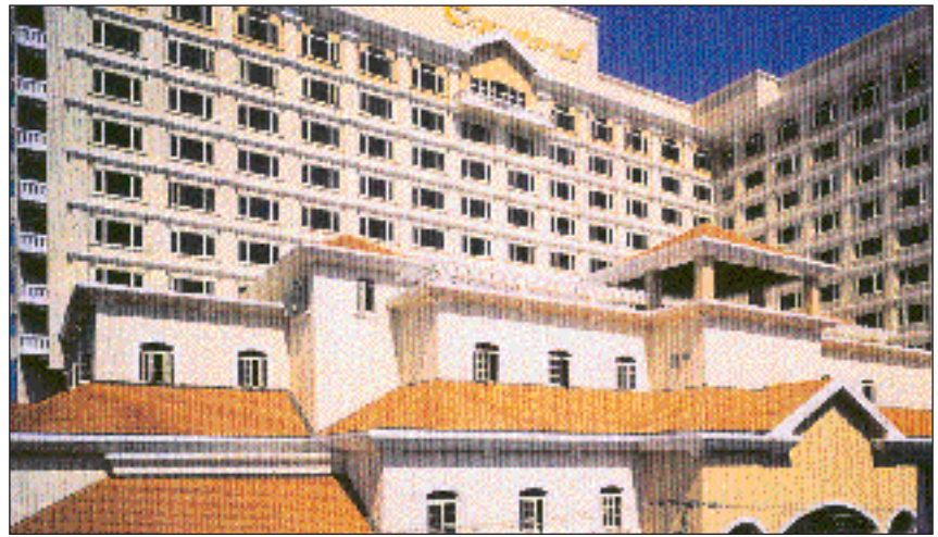
EQUATORIAL HOTEL FACADE WITH GRC FASCIAS, CORNICES AND COLUMN CLADDING.
