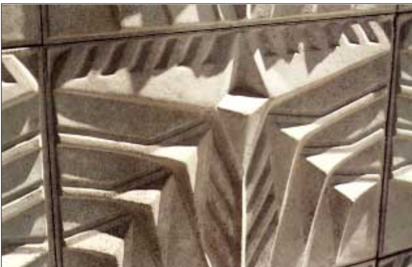
PHOTOGRAPH 3 USE OF AN ELASTOMERIC FORM-LINER. A VERY EXTENSIVE RANGE OF PATTERNS IS AVAILABLE.
