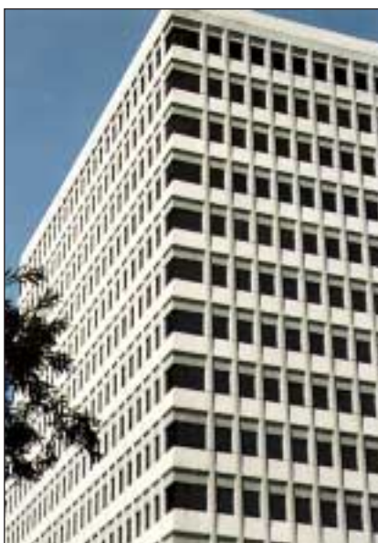
PHOTOGRAPH 6 THE NEAR PRISTINE APPEARANCE OF WATER-WASHED FACADE, NOW AROUND 20 YEARS OF AGE.
