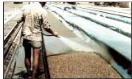
PHOTOGRAPH 8 WASHING OPERATION. IN THIS INSTANCE, APPLIED TO HOLLOW CORE PLANKS.
