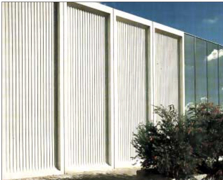
PHOTOGRAPH 1 SMOOTH, RIBBED FINISH USING AN OFF-WHITE CEMENT.
