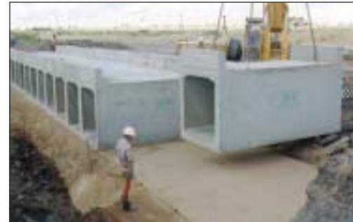
15.30 HOURS SUNDAY PENULTIMATE UNIT BEING LOCATED
