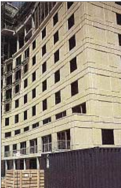
A QUALITY CLASS 2 FINISH, AIDED BY GOOD ARCHITECTURAL DETAILING (Courtesy Sydney Harbour Casino Pty Ltd)
