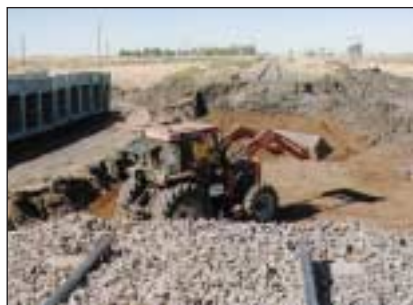
10.00 HOURS SUNDAY SUB-BASE PREPARATION
