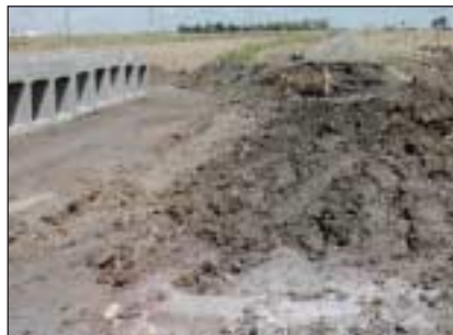
17.00 HOURS SATURDAY ONGOING SITE CLEARANCE
