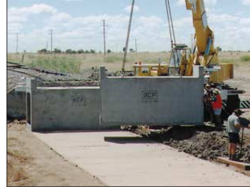
14.00 HOURS SUNDAY BASE COMPLETED, UNITS BEING PLACED
