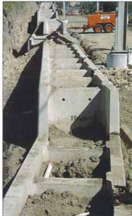
'DOUBLEWALL', EARTH-FILLED RETAINING WALL SYSTEM.
