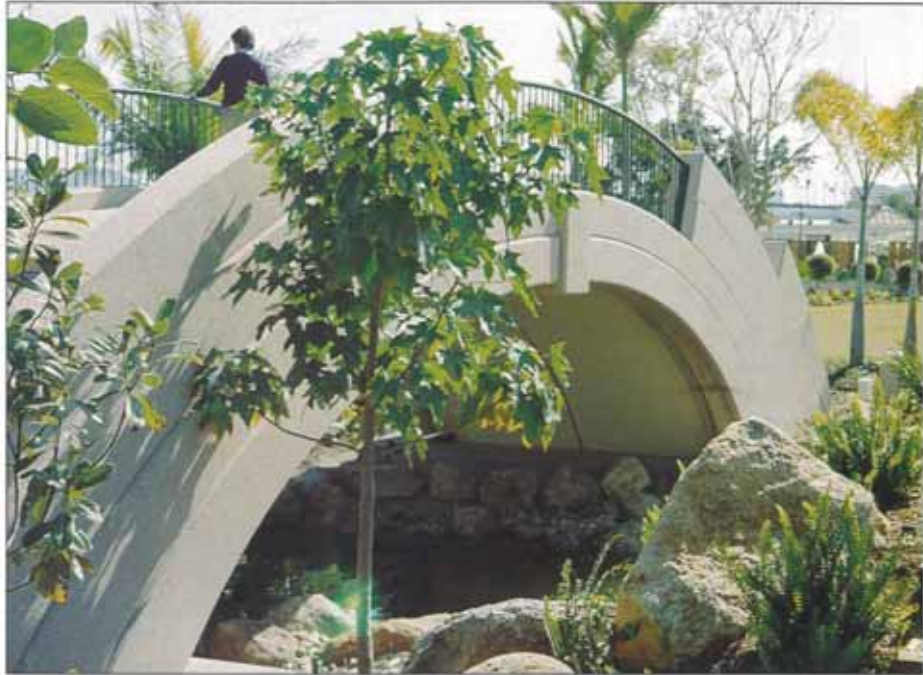
BEBO ARCH USED AS A PEDESTRIAN FOOTBRIDGE PROVIDING PLEASING AESTHETIC LINES.
