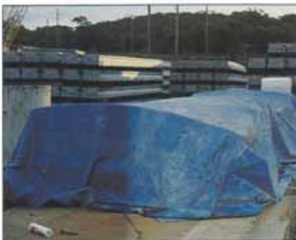
HEAVY DUTY TARPAULIN PROVIDING CURING ENCLOSURE TO PRECAST, PRESTRESSED BRIDGE BEAMS
