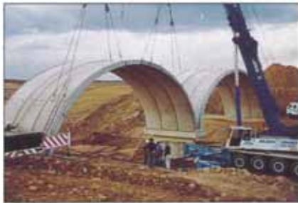
CLASSIC ARCH UNITS BEING ERECTED – PENRITH LAKES BRIDGE, OLYMPICS 2000 ROWING COURSE.
