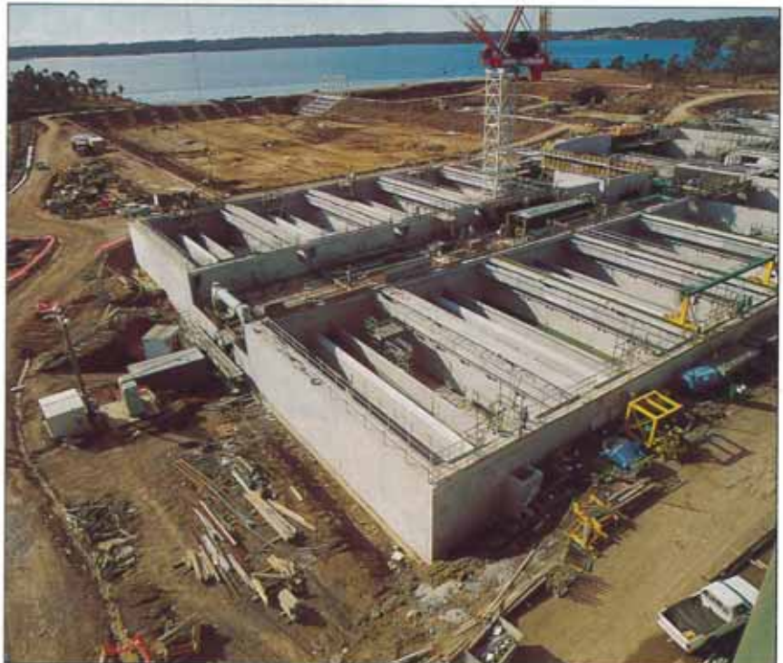
OVERALL VIEW OF THE FILTERING CHAMBERS
