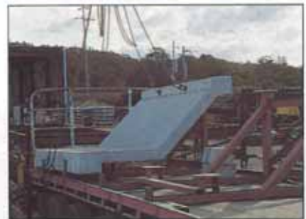
PRECAST LAUNDRER UNITS BEING LIFTED FROM PURPOSE-MADE TRANSPORTING FRAME
