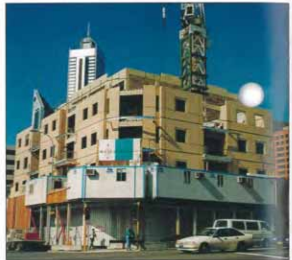
FULLY PRECAST, TERRACE STYLE HOUSING, NORTH ADELAIDE
