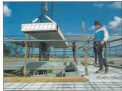
PLACING HOLLOW CORE FLOOR PLANKS.
