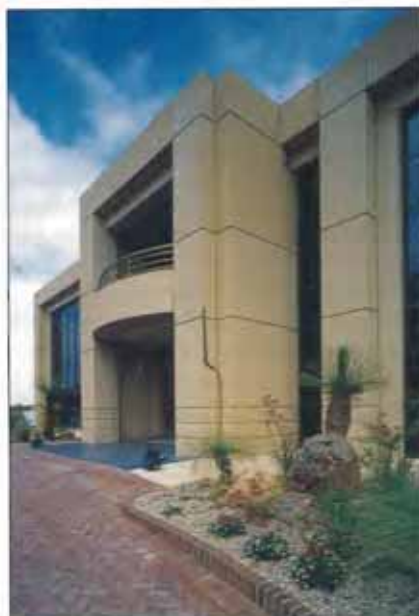
CLASSICAL FACADE, BEIERSDORF AUSTRALIA LTD. SANDBLASTED FINISH WITH FEATURE AREAS SUCH AS WINDOW SURROUNDS POLISHED. (BY RESCRETE)
