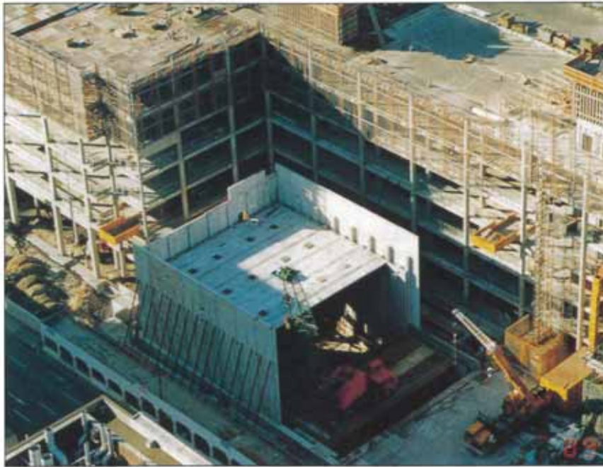
ABC STUDIOS SYDNEY: ERECTION OF THE EUGENE GOOSSENS RECORDING HALL (A DOUBLE-SKIN WALL AND ROOF ARRANGEMENT USING SINGLE TEE UNITS), INNER ROOF BEING PLACED ON INNER WALL SKIN.
