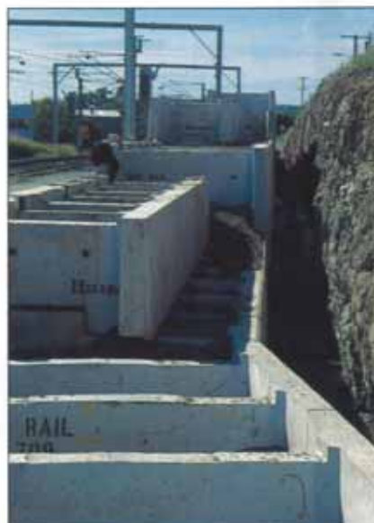
■ DOUBLEWALL CONSTRUCTION IN PROGRESS
