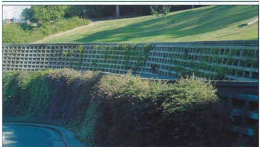
■ CRIB WALL – EFFICIENT AND VISUALLY PLEASING
