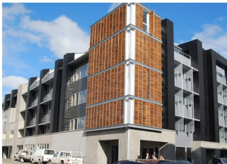
Victorian precast concrete manufacturer Hollow Core Concrete supplied 4,600 square metres of hollowcore precast flooring planks to the 5-storey building. Apart from the ground floor being in in-situ concrete, all remaining floors were in hollowcore to eliminate the need for expensive and time-consuming formwork.
