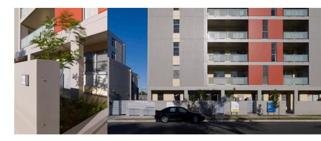
horizontal reglets define each storey and rich red panels are separated by a neutral band at each floor. All this was achieved through careful coordination and communication between architects, precast manufacturers and builders during construction, expediting and streamlining construction, whilst maintaining the integrity of the design intent.
