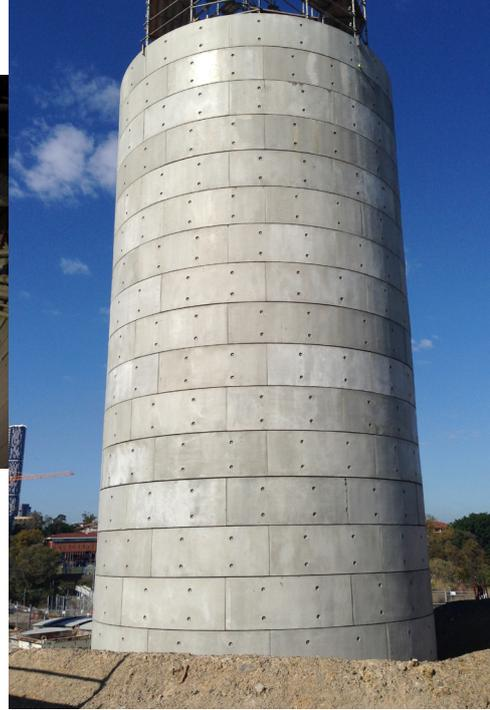
By taking advantage of strength and durability of precast concrete, the asset owners were provided with a storm water management system with a certified design life of 100 years.
