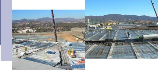
The tight fast track construction programme set by Multiplex required that the installation of the floors was a critical element. Ultrafloor were able to respond by each week installing up to 5,000 square metres of flooring. That's the equivalent of a massive 50 house floors in area. The Ultrafloor requirement was for six levels of suspended precast concrete flooring, amounting to 50,000 m2 GFA in total.
