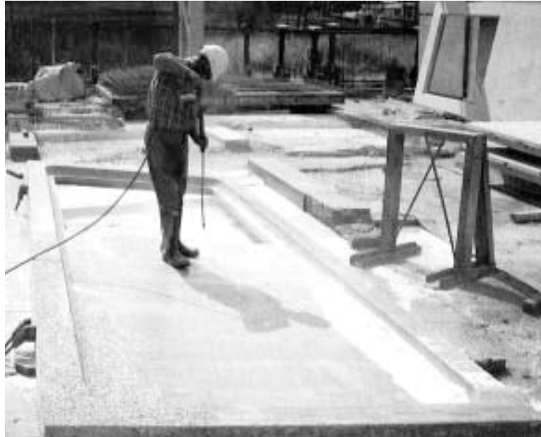
Facing page: top – example of vertical casting to obtain a smooth off-form finish on both sides; middle – aggregate exposed by water-washing in the casting yard; bottom – water-washed aggregate finish.
