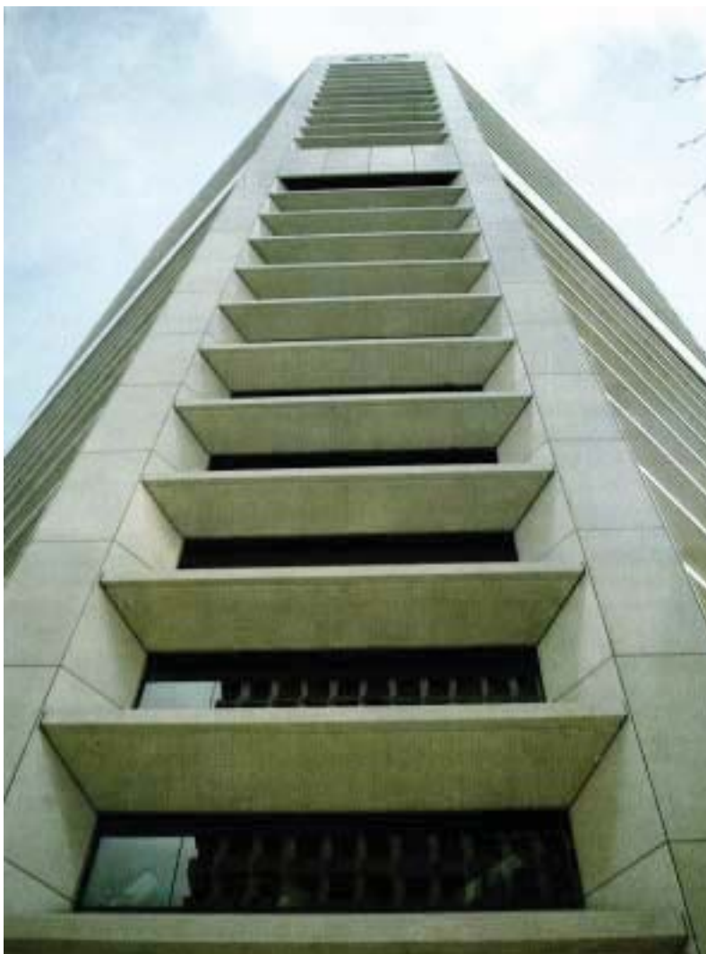
Facing page: top left – Wet sandblasting of striated finish; bottom – spandrels with striated finish; top right – offices, Mary Street, Brisbane - sunhoods cast face down, then sandblasted.
