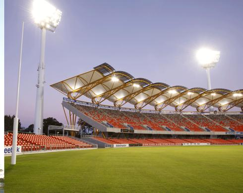
In total, more than 8,000 square metres of hollowcore flooring and a staggering 15 kilometres of seating were supplied by Precast Concrete Products.
