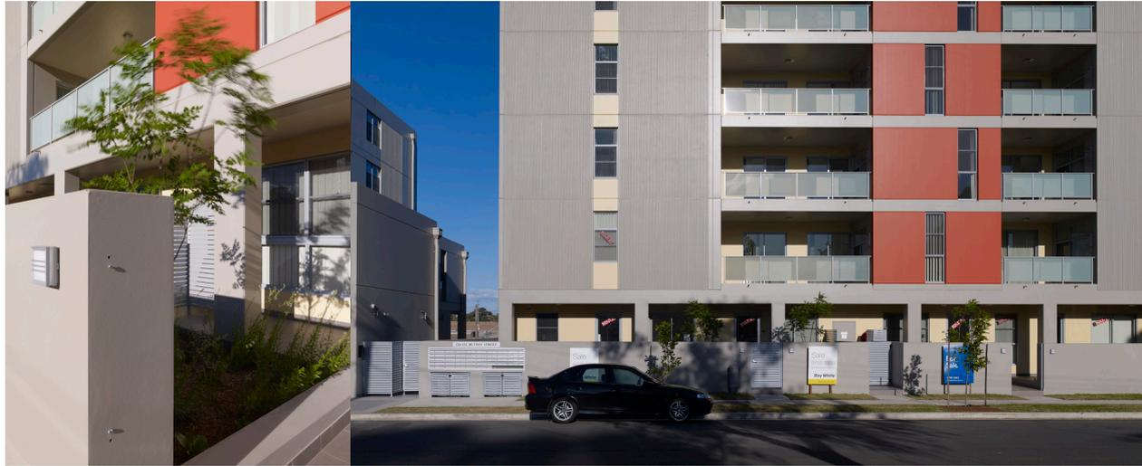
horizontal reglets define each storey and rich red panels are separated by a neutral band at each floor. All this was achieved through careful coordination and communication between architects, precast manufacturers and builders during construction, expediting and streamlining construction, whilst maintaining the integrity of the design intent.
