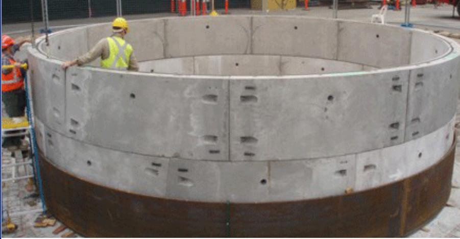
The WDA sub-contracted Humes to supply and design the proposed shafts, who then in turn engaged Halcrow to check the segmental linings, design the shaft and all temporary works for the shaft construction process, and provide details for openings in the lining to receive the tunnelling machine being jacked from another shaft. Both of the temporary shafts were designed with a 7.5m internal diameter and measured 12 to 15 metres deep.
