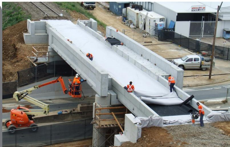
To maintain the existing rail level, a modified precast cross deck section was conceived, with use of 8 no. 1200mm diameter bored piles located outside the existing bridge structure, along with cast in situ columns to form the sub-structure. The headstocks and abutment beams were cast as high as possible under the existing bridge, while concrete packing beams gave the new bridge greater clearance.
