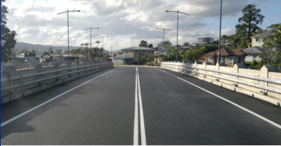
Humes delivered a tailor-made decorative precast solution to ensure the new bridge faithfully represented the art deco style. Specially made moulds were used to create the 108 decorative precast plinths and 112 decorative precast infill panels. As well, 12 precast arch facades were supplied, the spans of which were built to imitate the original arches. All elements in the new Jubilee Bridge met stringent load standards set down by the Queensland Department of Transport and Main Roads.
