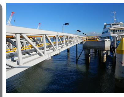
for the in-situ concrete to bond to. The dolphins are supported on steel piles driven into the sea bed. Use of both dolphins and piers enables the overall size of the piers to be considerably condensed.
