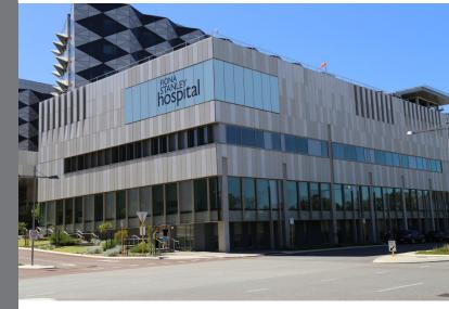
Each of these structures features extensive use of architectural precast walls and Deltacore™ floor planks, supplied by Delta Corporation. Precast was chosen because it offers architectural finishes of various colours and textures that can't be achieved with conventional construction.
